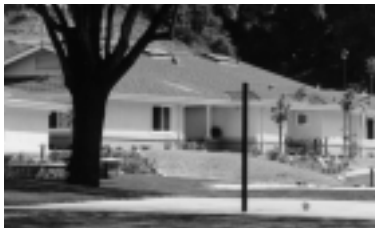
Located in the upper campus of Hillside, two new cottages were built to house ten children each. Adjacent to these homes are a playground and pool for cooling off during the summer months.
